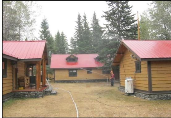
Figure 6. Firefighter testing a tripod mounted sprinkler.
