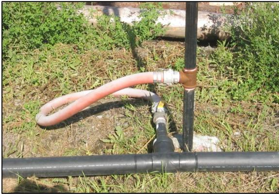
Figure 3. The connection from the high-density polyethylene supply line to the sprinkler.
